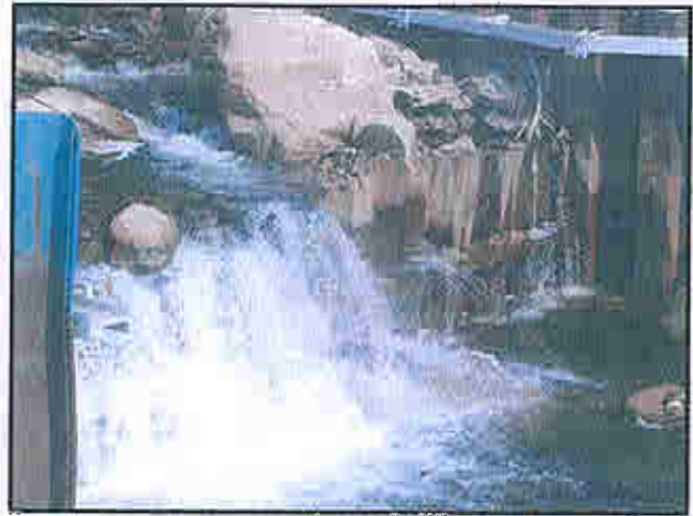
The weir at the lower bridge (above) before 2005. Photo courtesy of Imperial Oil Resources Limited.
