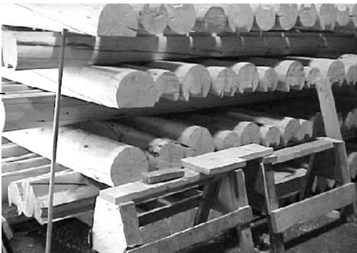
COMPLETED WALL LOGS scribed, grooved and oiled, and ready for final assembly.
