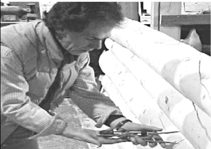
SCRIBING is the most important step. The log is scribed using a bubble-level on both sides.
