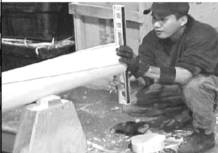
A PLUMB LINE at both ends of the log is traced from the centre line.
