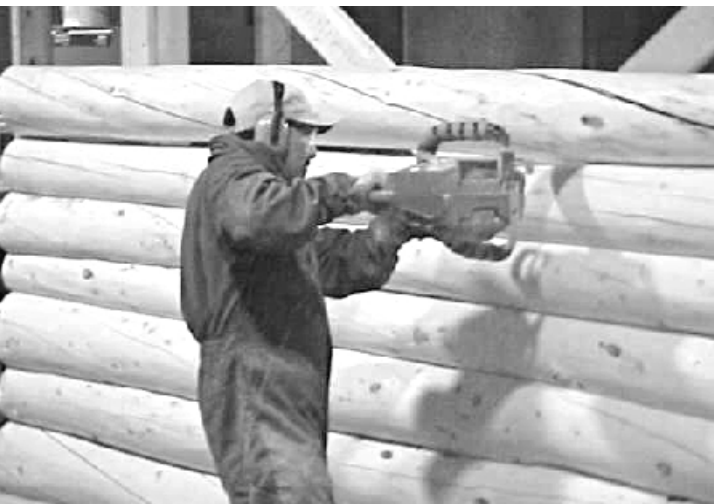
PRIOR TO SCRIBING some logs require chain saw cuts to eliminate high spots, making the log sit more level.
